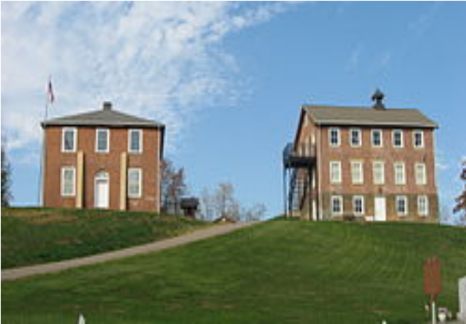
The Old Chester Courthouse and Academy - Chester, Ohio
